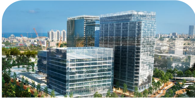
RISHO Complex Rishon LeZion 190 thousand m 2 | US$ 269 million
