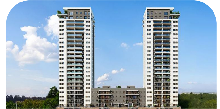
Ashtrom Park Be'er Ya'akov** 260 Units
